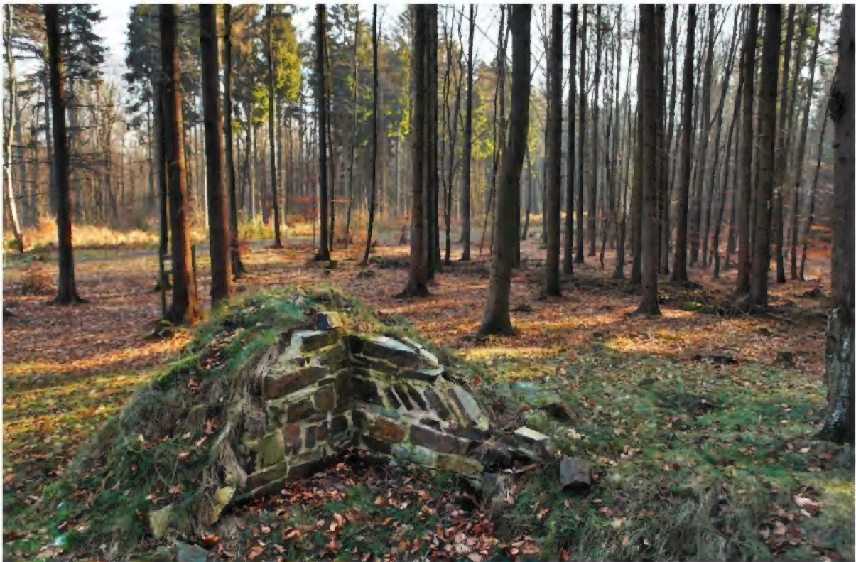
BEHELN, GERMANY Only a few stone foundations remain from the more than 800 watchtowers built by Roman soldiers along 342 miles of the frontier linking the Rhine and Danube Rivers.
